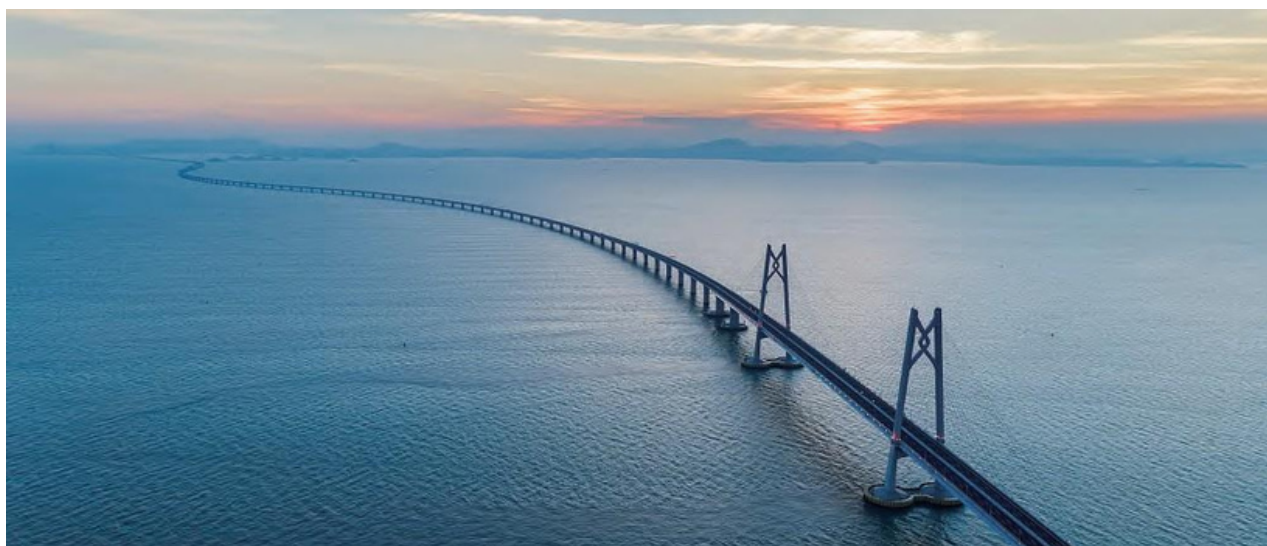
Application during major port construction
